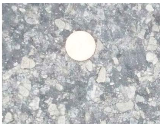
Roadway surface, asphalt concrete ACo roadway surface 11 - 15 years old (on the right)
