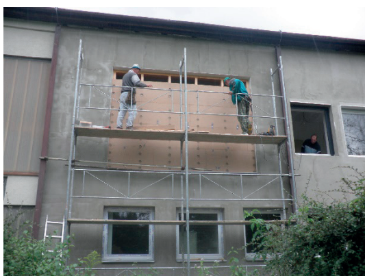
Fig. 3 Montage of MDF board (September 2010)
