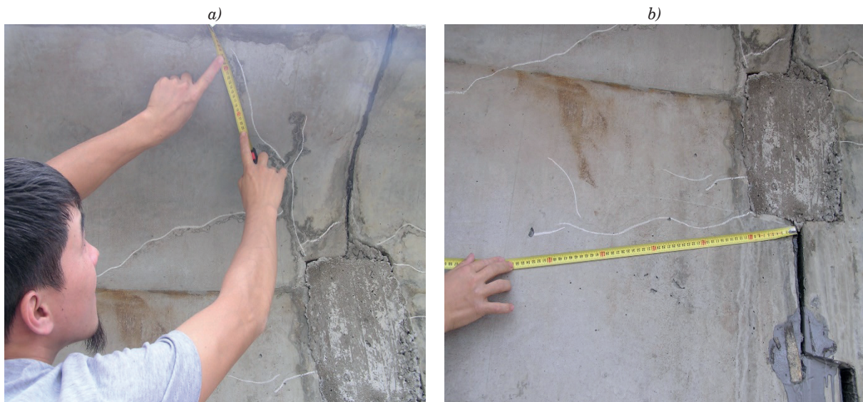
Figure 12 Cracks formation in blocks concrete in the monolithic insert zone after stressing of 42.0 m-long composite beam by tendons: the southern side of No. 1 adhesive joint; b) the northern side of No. 1 adhesive joint
