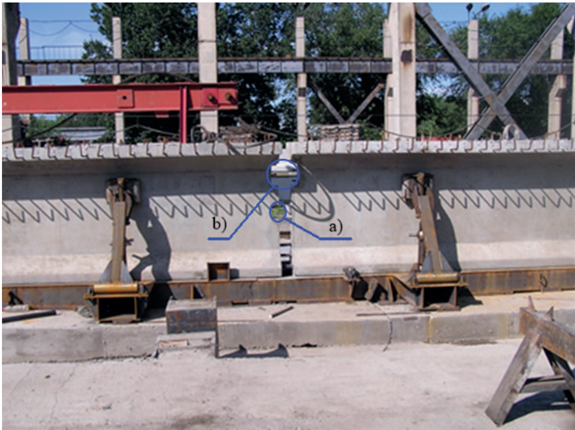
Figure 5 No. 2 adhesive joint zone (the middle segment on the left in the picture): there is a “tooth” and a “cutout” for the formation of a dowel in the middle part of the height of segments, b) “cutouts” are placed in the upper zone of the segment edges, to form a monolithic dowel
