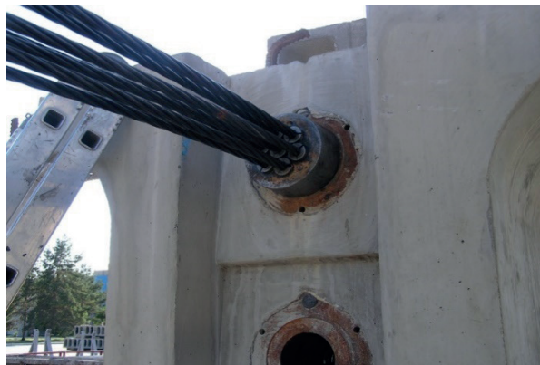
Figure 8 K-7 Ø15 anchored strands of the upper tendon
