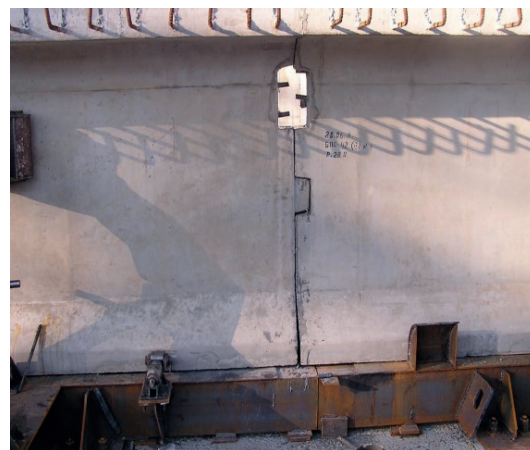
Figure 9 Missing contact of the segment heads of 42.0-m-long composite beam in No. 1 adhesive joint zone after the tension of the prestressing tendons
