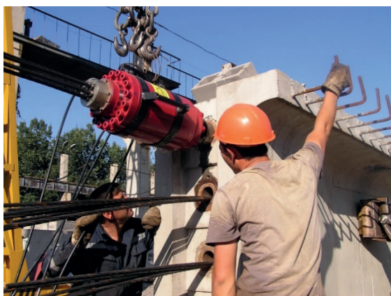
Figure 7 Tension of the upper tendon made of K-7 Ø15 strands
