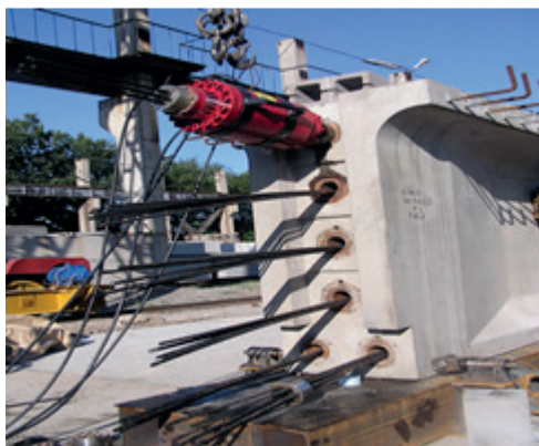
Figure 6 General view of the end face of the outer segments with K-7 strands laid in channel formers, a hydraulic jack is installed at the top for tensioning the upper due to prestressing tendons
