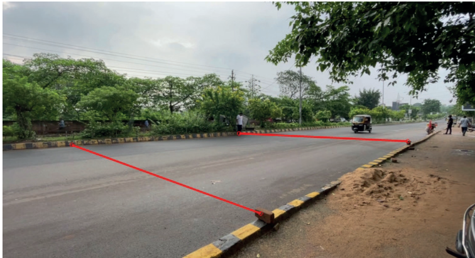
Figure 1 Snapshot from one of the sites illustrating the temporary road markings
