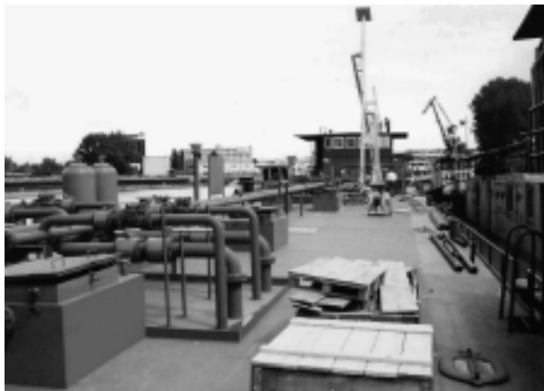
Obr. 6 Prestavba lode Fig. 6 Rebuilding of the ship
