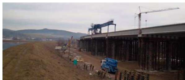
Fig. 7 Construction of the highway bridge 207
