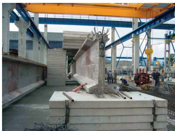
Fig. 3 The test setting up
