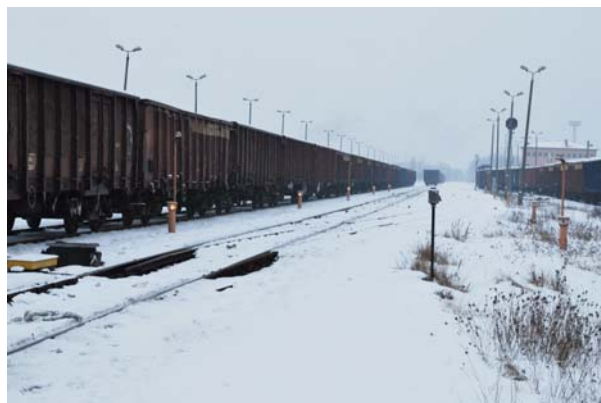
Fig. 5 Unloading rail tracks
