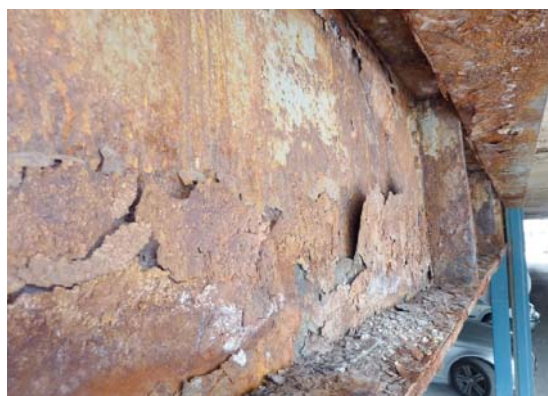
Fig. 3 Views of the steel frame details of the external car park roof structure (the condition before the renovation)
