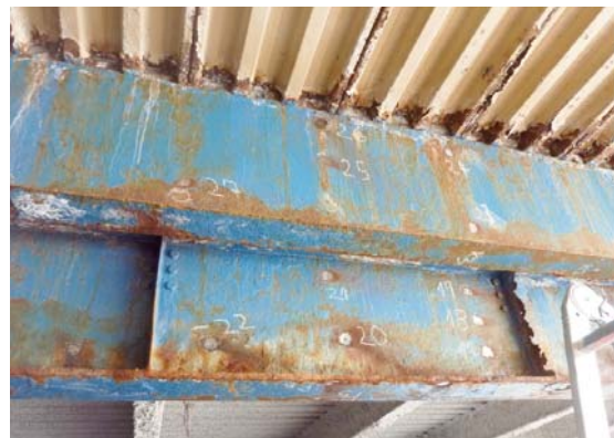
Fig. 2 Experimental measurements of the section thickness of Beam 6 in the most exposed locations
