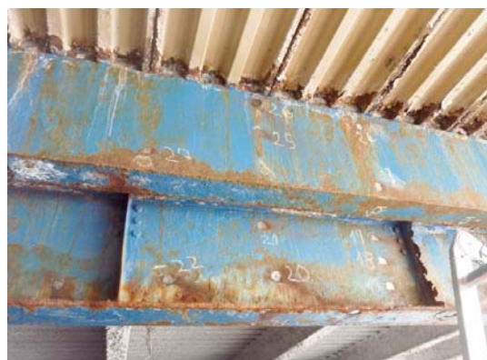
Fig. 3 Views of the steel frame details of the external car park roof structure (the condition before the renovation)
