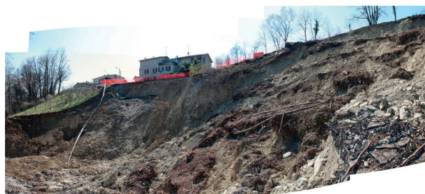
Fig. 3 Boschetto landslide's crown area. The provincial road that crossed the slope just in front of the depicted house was completely destroyed by the landslide, causing the seclusion of the inhabited upper Parma river valley
