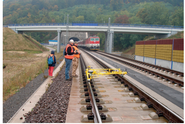
Fig. 1 Type of Ballastless Track Construction RHEDA 2000
