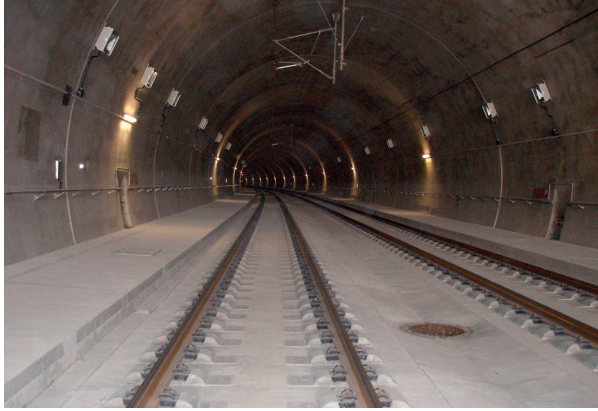
Fig. 1 Type of Ballastless Track Construction RHEDA 2000
