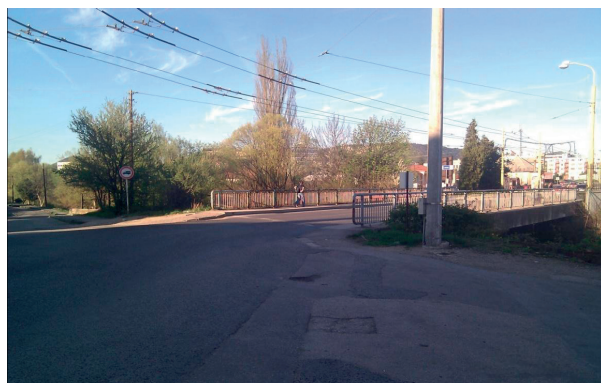
Fig. 2 Chosen bridge [authors]
