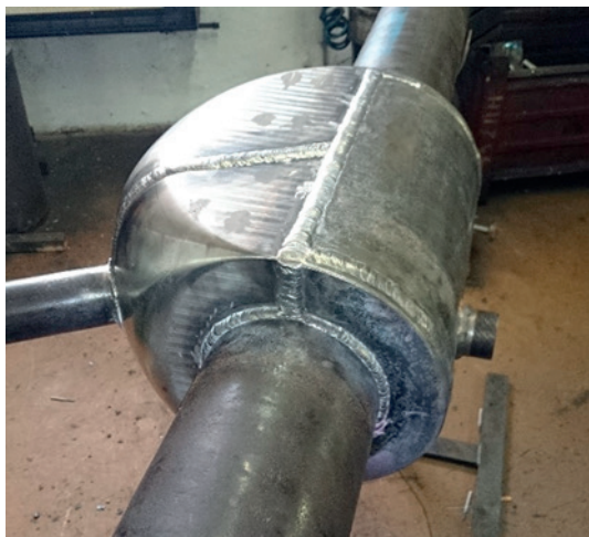
Fig. 1 Split sleeve for branch connection repairs
