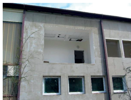
Fig. 1 Beginning of construction work on the laboratory - prepared opening for wooden frame (April 2010)
