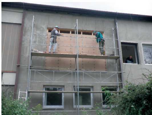
Fig. 3 Montage of MDF board (September 2010)
