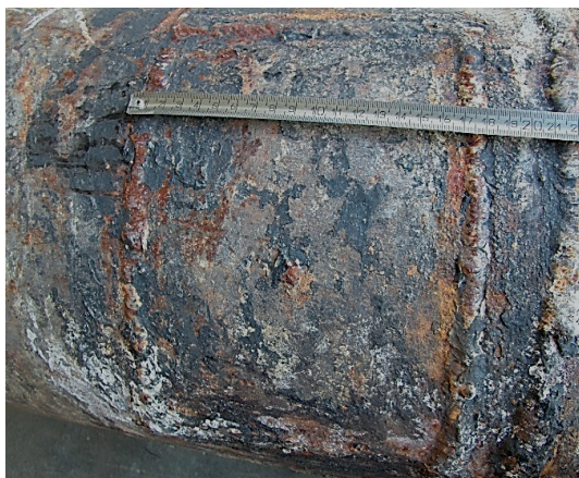
Figure 1 Steel repair-patch A
