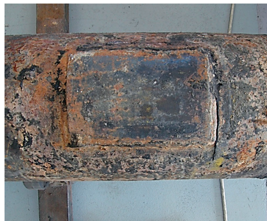
Figure 2 Steel repair-patch B
