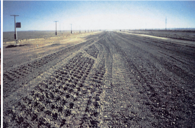
Figure 5 General view of the crushed asphalt scrap padfoot roller
