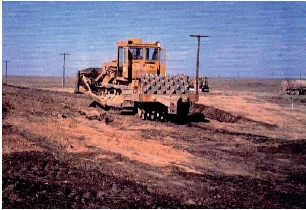
Figure 4 Cam roller with opening of the asphalt concrete pavement
