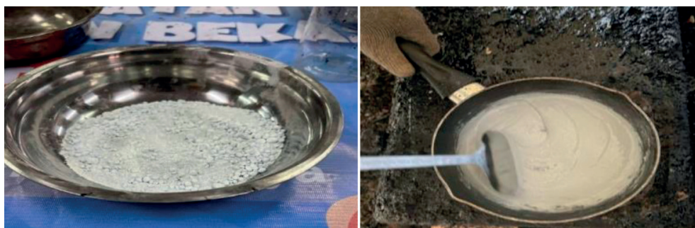
Figure 2 Phosphorus addition to road marking paint and heating of thermoplastic paint
