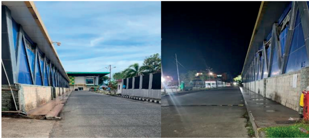
Figure 1 Condition of sidewalk at UNP campus
